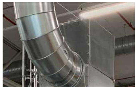
Quick-Fit Segmented Bends allow airflow direction change in a run of duct.
